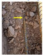
Rebar out of position to maintain 2" of concrete around all areas. Noted at both front corners of garage
