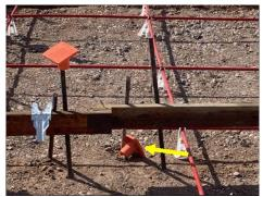
Clean all debris from area prior to Clean all materials from trenches Several safety caps not installed at form stakes
