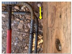
Rebar out of position to maintain 2" of concrete around all areas. Noted at both front corners of garage
