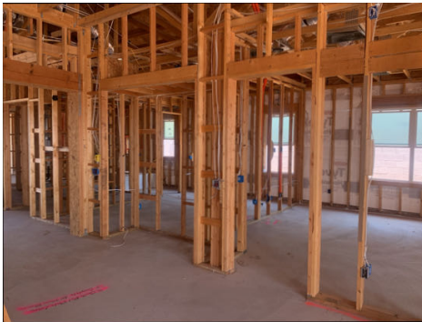
General view of home
