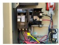
Wiring improperly doubled at pool sub panel
