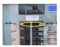
Two upper 20 amp circuit breakers were tripped. Reset OK. For outlets below panel.
