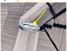
Cracking or separations noted at mortar flashings at rear roof hip
